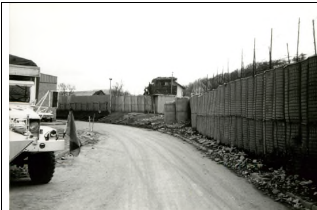
View of the earthen walls that were erected around the base to provide more protection. Frames of hessian cloth are filled with earth Photo provided by Jacques Rioux
